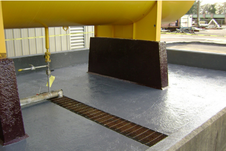
Belzona 4311 (Magma CR1) Epoxy novolac, high chemical-resistant barrier coating for concrete and steel protection.
