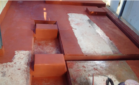
Belzona 4181 (AHR Magma-Quartz) Acid and heat-resistant epoxy concrete repair mortar.
