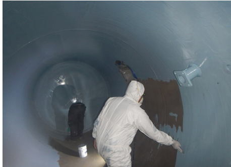
Belzona 1391T Hand-applied, high-temperature, abrasion-resistant epoxy coating for erosion-corrosion protection under immersion up to 130°C (266°F).
