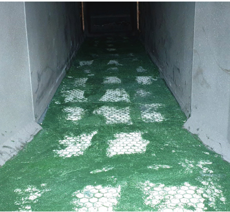
Belzona 1813 High-temperature, ceramic-filled abrasion and wear-resistant epoxy repair composite.
