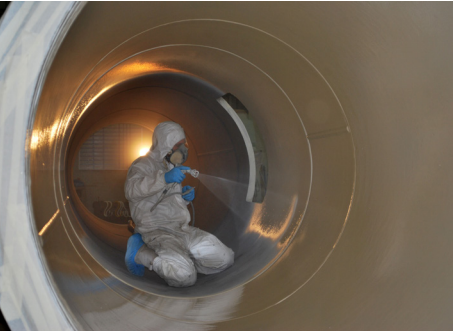
Belzona 1381 Sprayable, erosion-corrosion-resistant epoxy coating with ultra-high molecular weight polymer fillers for immersion up to 95°C (203°F).
