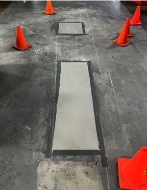
Belzona 4111 (Magma-Quartz) A magma-consistency repair/rebuilding system for repairing and resurfacing concrete and stonework.
