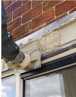
Belzona 4141 (Magma-Build) Lightweight epoxy concrete repair mortar suitable for vertical and overhead applications.
