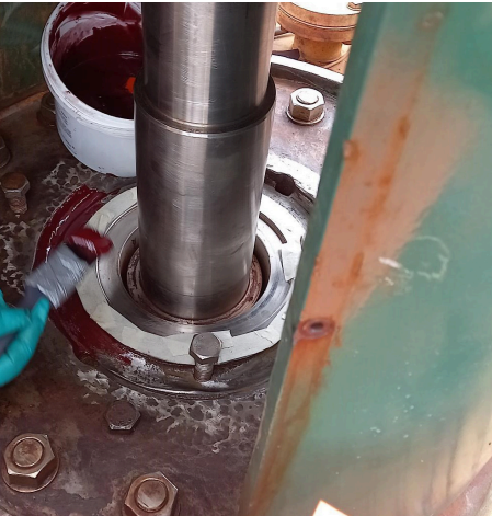
Belzona 4331 (Magma CR3) Epoxy novolac barrier coating for concrete and metal protection, offering high resistance to hot organic acids.
