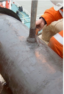
Belzona 1251 (HA-Metal) High-performance, heat-activated epoxy repair composite for applications directly onto hot metal surfaces.
