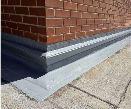
Belzona 3121 (MR7) Emergency repair and waterproofing system for sealing all types of surfaces and structures against atmospheric attack.
