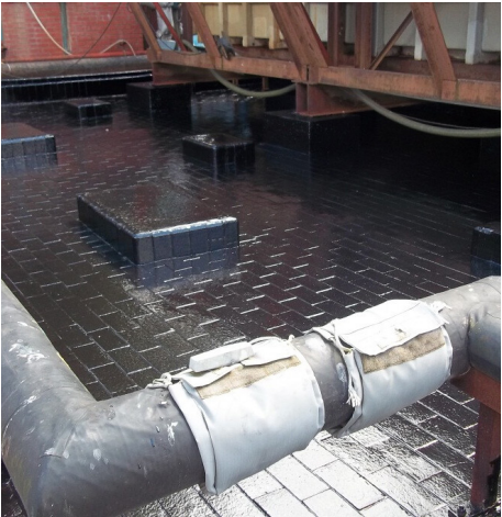
Belzona 4351 (Magma CR5) Epoxy novolac, static-dissipative barrier coating suitable for concrete and metal protection, offering high resistance to a broad range of chemicals.
