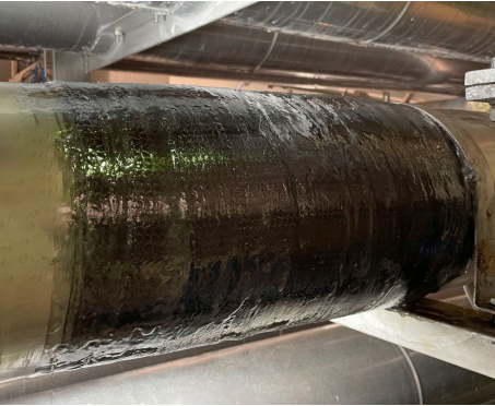
Belzona 1983 High-temperature resin for application temperatures of 5°C (41°F) - 40°C (104°F) and operating temperatures up to 150°C (302°F).
