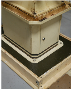
Belzona 7211 A high strength, low exothermic, 100% solids, low VOC system for deep pour grout. Sold exclusively in the Americas.
