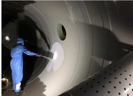
Belzona 5892 Epoxy barrier coating suitable for surfaces in contact with aqueous solutions at temperatures up to 95°C (203°F).
