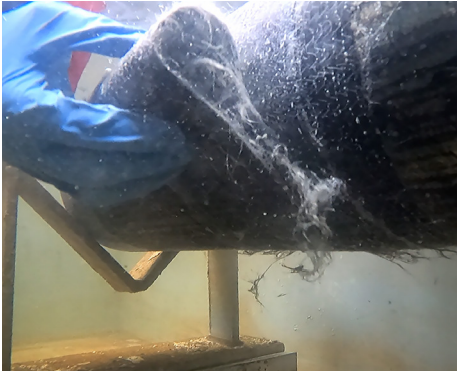
Belzona 1984 Surface tolerant resin for service temperatures up to 50 °C (122 °F) and suitable for minimum application temperature of 5 °C (41 °F).
