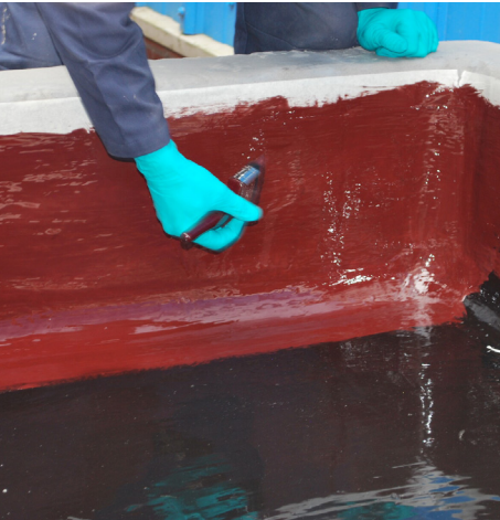
Belzona 4361 Flexible chemical-resistant epoxy barrier coating suitable for concrete protection. Particularly suitable for areas subject to movement.
