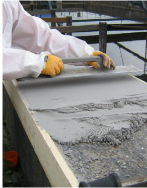
Belzona 4131 (Magma-Screed) Epoxy impact and abrasion-resistant concrete repair mortar.
