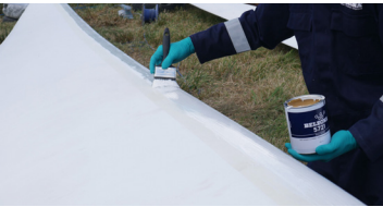
Belzona 5721 High-performance, solvent-free coating system specifically developed for protecting the leading edges of wind turbine blades from erosion and impact damage.
