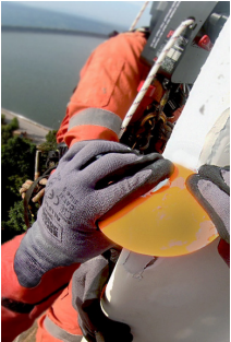
Belzona 5711 High-performance, solvent-free rebuilding material for repairing damage to the leading edges of wind turbine blades.
