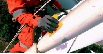
Belzona 5711 High performance, fast curing system for the repair of erosion and impact damage on leading edges of wind turbine blades.
