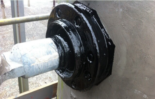
Belzona 2111 (D&A Hi-Build Elastomer) Flexible rebuilding-grade abrasion-resistant polyurethane elastomer, suitable for repairing damaged rubber and metal surfaces.
