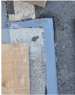
Belzona 4521 (Magma-Flex Fast curing, cost-effective flexible sealant suitable for construction and expansion joints on horizontal porous substrates such as concrete.
