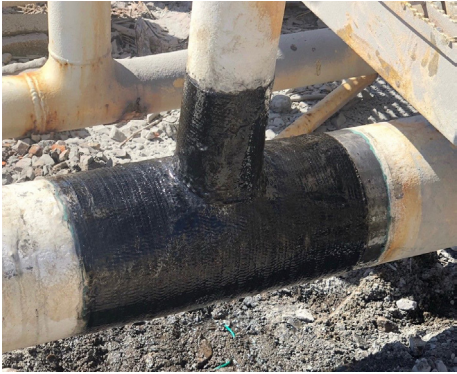
Belzona 1982 Extended working life resin for application temperatures of 20°C (68°F) - 40°C (104°F) and operating temperatures up to 80°C (176°F).
