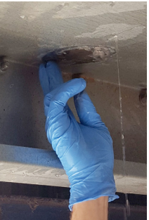
Belzona 9611 Rapid-curing system for the emergency sealing of low pressure leaks, prior to a more permanent repair.
