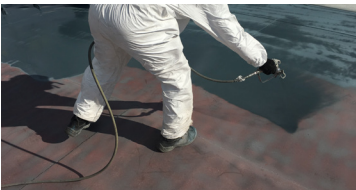
Belzona 6111 (Liquid Anode) Zinc-rich epoxy coating suitable for providing long-term galvanic protection to metallic surfaces.
