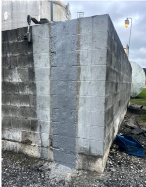
Belzona 4124 (Bulkfill) A cost-effective rebuilding system for repairing large volumes of concrete and stonework subjected to mechanical and chemical damage. Sold exclusively in the Americas.
