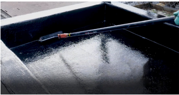
Belzona 5813 Solvent-free, cost-effective static-dissipative barrier coating designed to transfer the build-up of electrostatic charge away from hazardous areas.
