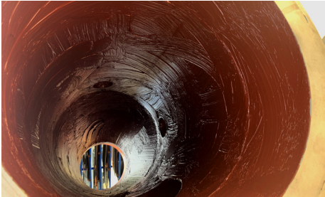
Belzona 4301 (Magma CR1 Hi-Build) Highly chemical-resistant epoxy novolac repair and resurfacing composite.
