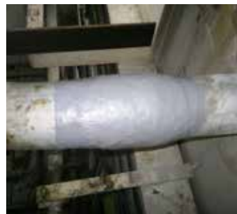
Wrapping and patching
