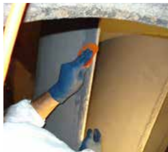
Forming and rebuilding
