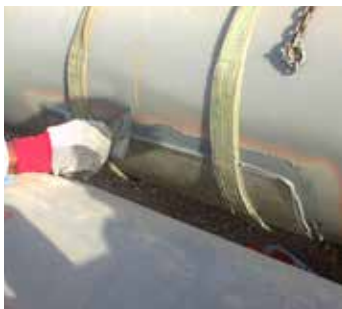
Bonding and shimming
