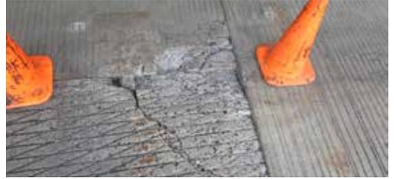
A concrete panel had cracked causing problems on the road
