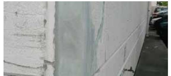
Belzona 4151 was injected before cracks were filled with Belzona 4111
