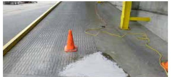
The Belzona 4151 + 4111 system was used to rebuild and smooth the cracked area
