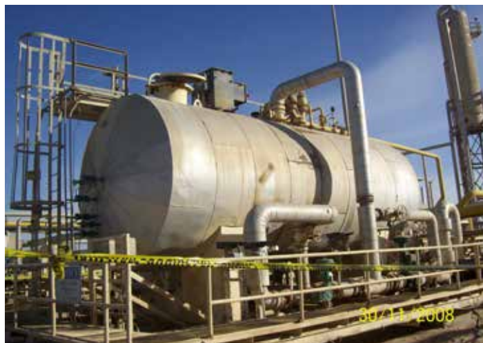
Belzona 5892 used to line a desalter
