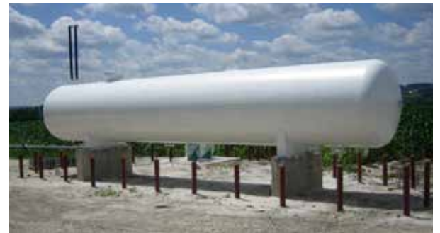
Completed application using Belzona 5111 for further protection
